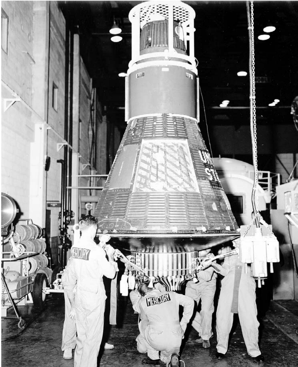
Figure 9.8. The Mercury capsule. The spherical heat shield can be seen as can the shingles on the upper body. Courtesy NASA.
